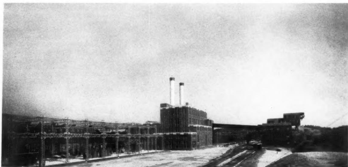
Duke Power Company's new Cliffside generating plant, typical of dozens of new plants just completed or under construction. This constant expansion of facilities to render
